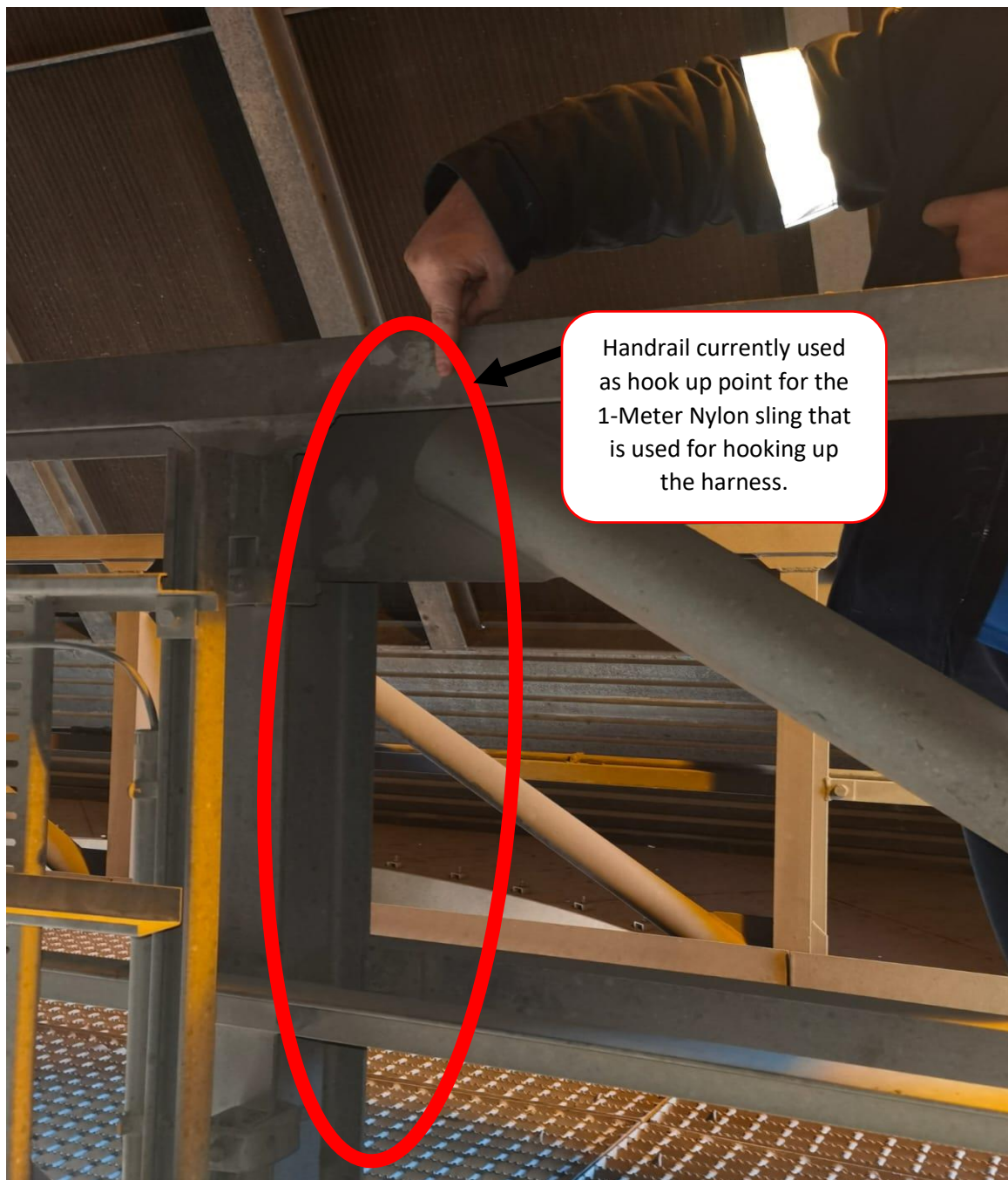
Figure 1. Nylon Sling Connection.
